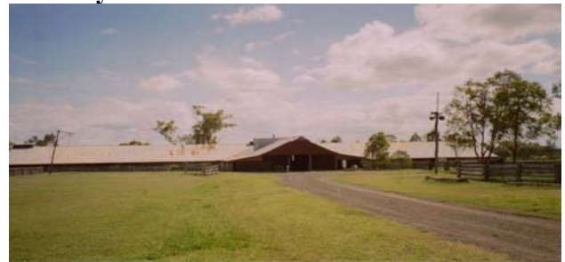
Jondaryan Barn built in 1853 still in excellent condition.
